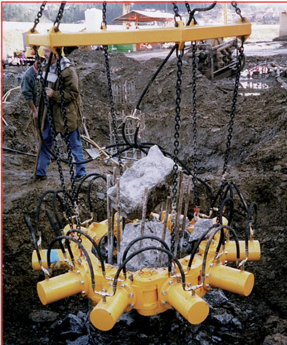
The pile breakers type 314 and 380 are highly modular systems that are easy to adjust to each pile diameter at site.
