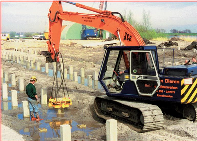
New series hydraulic pilebreakers for square piles.
